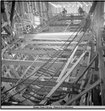
Construction of Princeton-Hall, Howard bros. shop, Katlian St. Image from Alaska State Library
