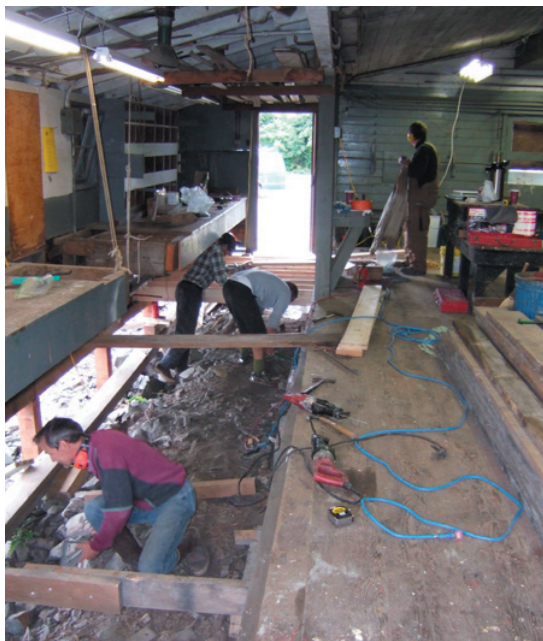
Replacing joists in workshop addition, summer 2006.
